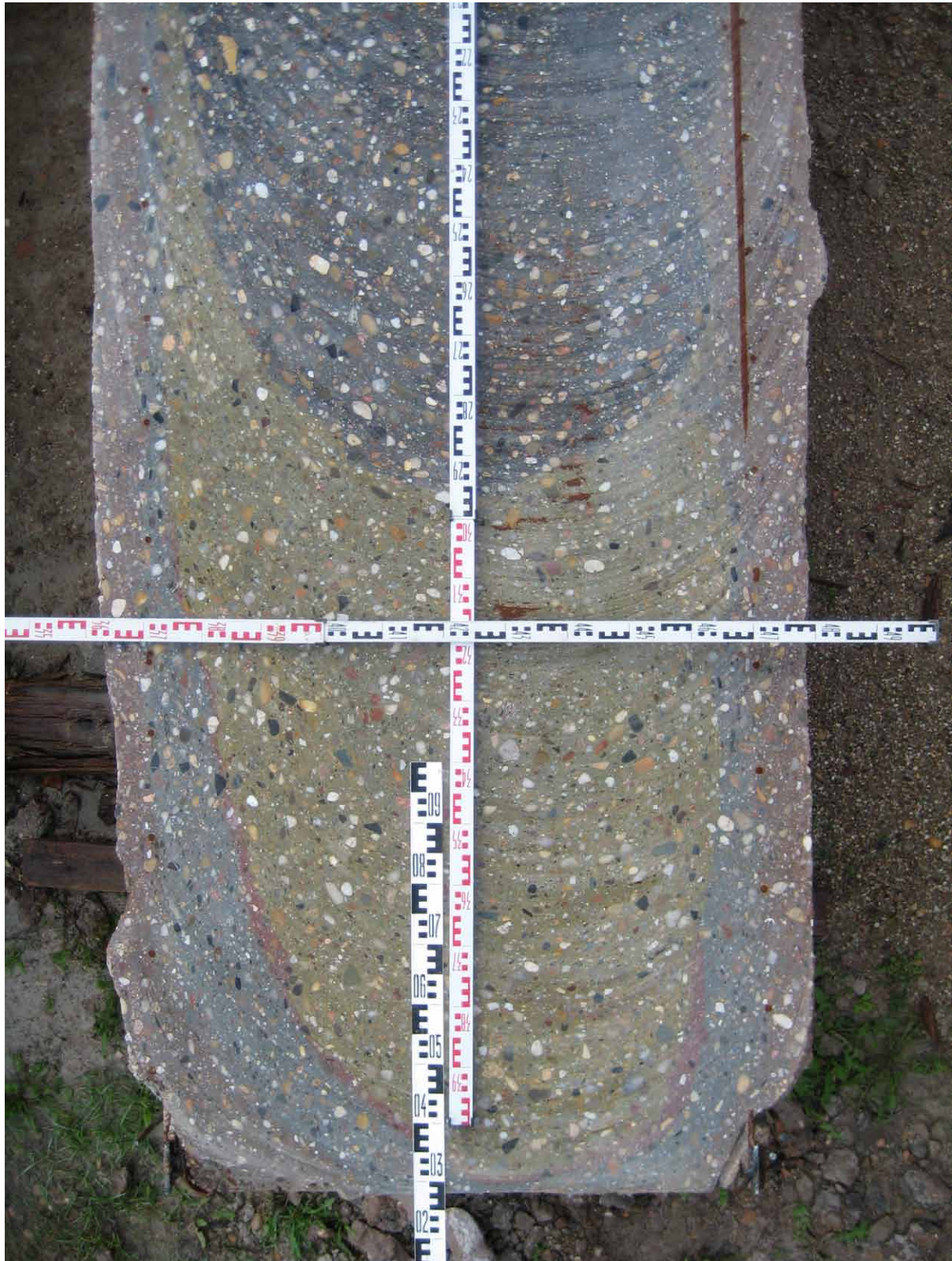
FIGURE 14: Cross section of a bored pile cast with differently dyed loads of tremie concrete (Böhle, Pulsfort, 2014)
