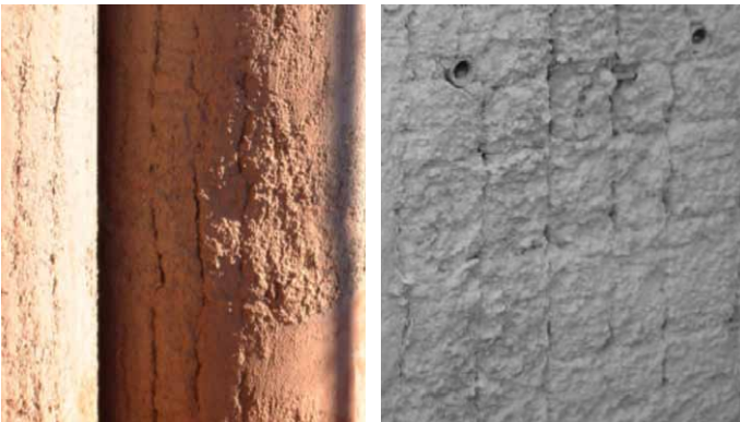
FIGURE E.4: Shadowing in a pile (left); mattressing in a panel (right)
